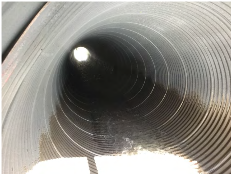
Roof and sidewalls from upstream
